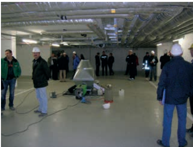
Smoke gas test preparation
